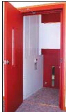
Fired rated steel door
